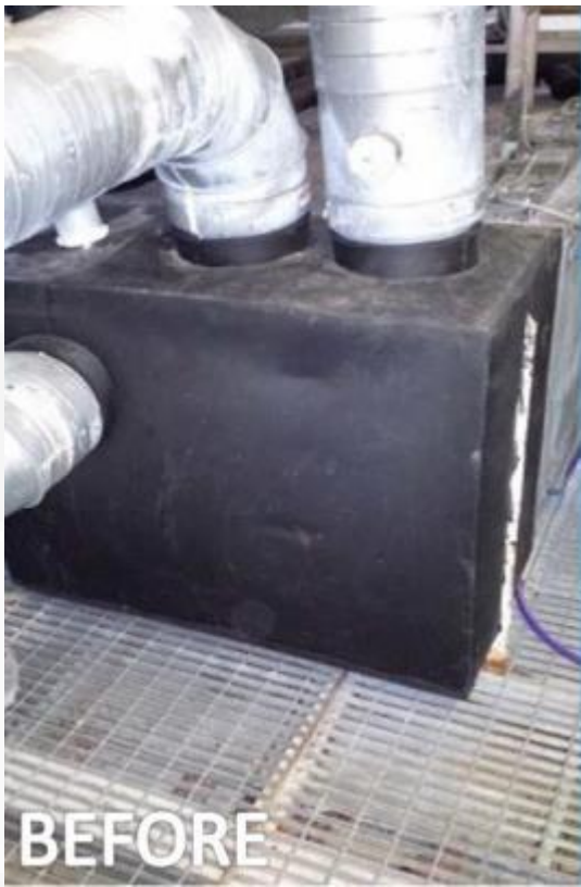
Insulated HVAC air conditioning plenum coming off air handling unit.
